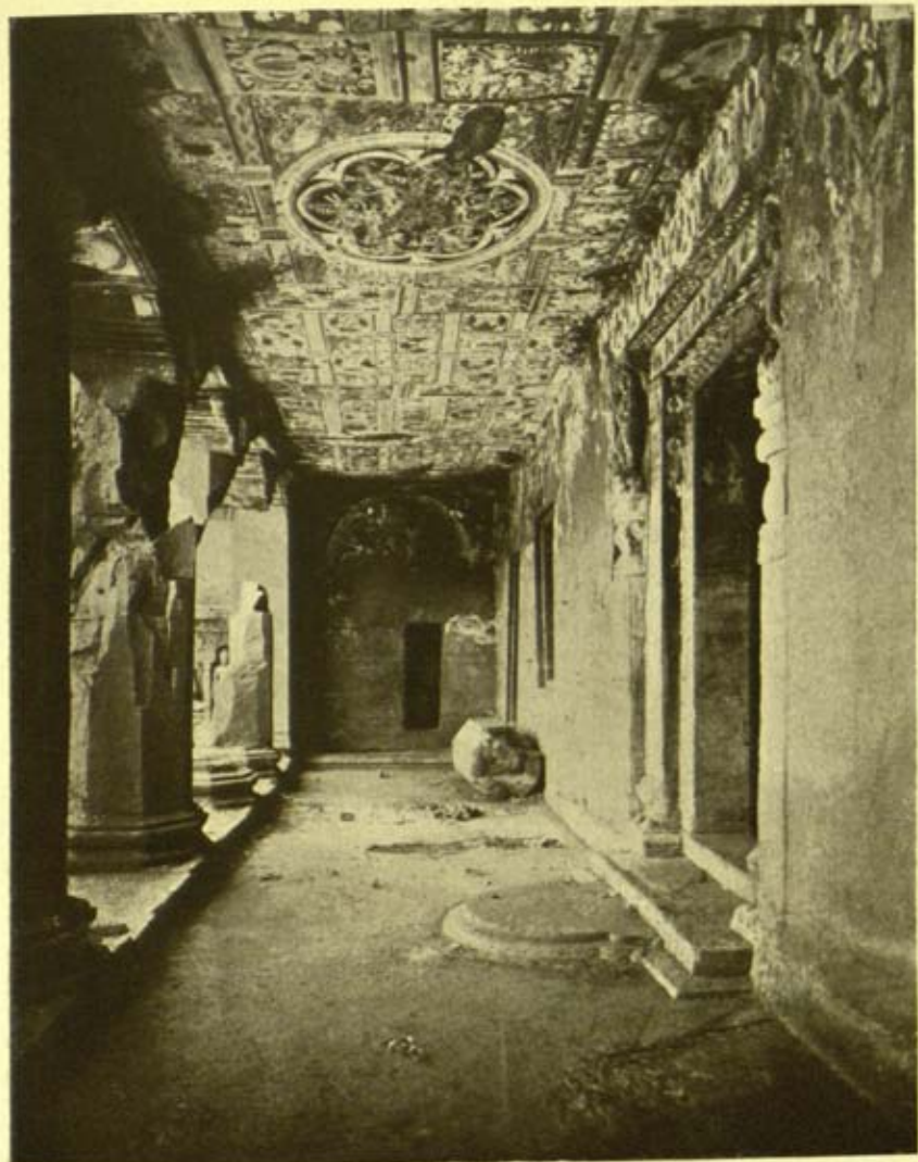
CEILING OF BARANDA. CAVE 17.
