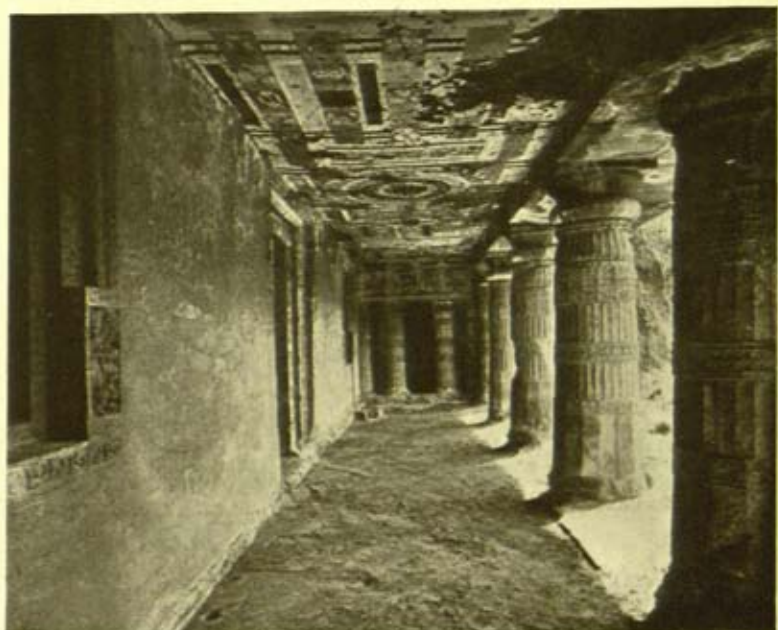
CEILING OF BARANDA.
